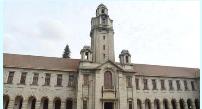
Indian Institute of Science building in Bengaluru
